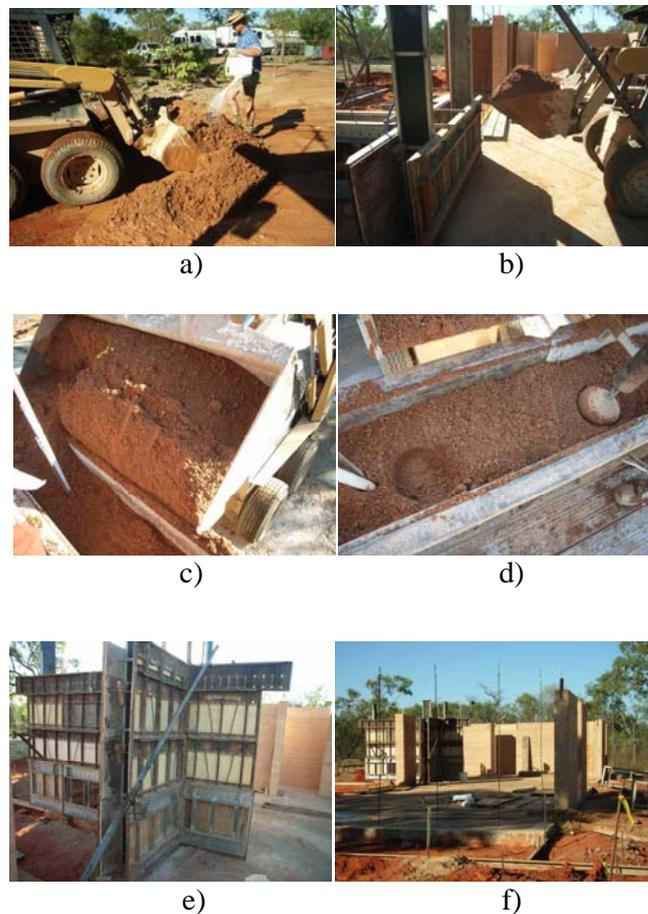
**Figure 1. Rammed earth construction procedure: (a) water is added to soil; (b) and (c) moist soil is put into the first layer of formwork; (d) moist soil is compacted; (e) following layers are built up in the formwork to achieve the desired height of the wall; (f) after 1 day the formwork is removed and the wall is allowed to cure**
